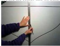
8. Measure on left & right, equal distance down, from top edge of boat to mark where bottom of vinyl boat letters will be. Draw horizontal line with Stabilo pencil.
