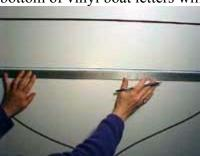
9. Tape the vinyl boat letters into position with masking tape, making sure to match horizontal and vertical lines.
